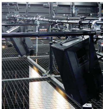
Meyer Sound UPQ speakers are affixed above the grid in the Black Box Theatre
