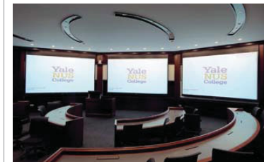
The three NEC NP PX750UG projectors and motorised Remaco screens in LT-60 receive their video signals from a Crestron DM1616 matrix whose inputs include Sony cameras, Blu-Ray players and PCs
